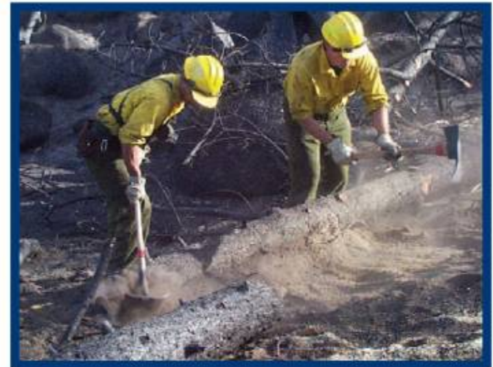
Figure 10.2—Installing contour-felled logs for erosion control after a wildfire. (Photoby Peter Robichaud).
